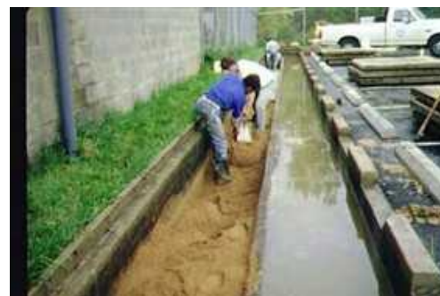
Routine cleaning of a perimeter or "Delaware" sand filter. This can be done from the surface, but deeper, vault-type filters will require confined-space entry procedures.
