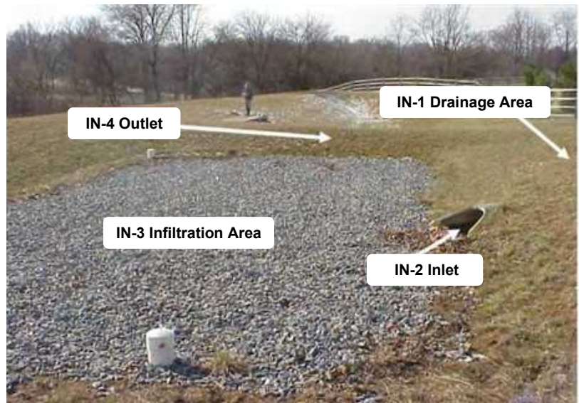
Figure 12.17 Key Areas for Level 1 Inspection of Infiltration Practices
