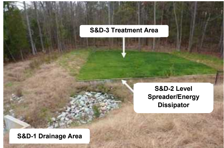
Figure 12.4 Key Areas for Level 1 Inspection of Sheet Flow and Disconnection with filter strip shown. (R. Winston, NCSU)
